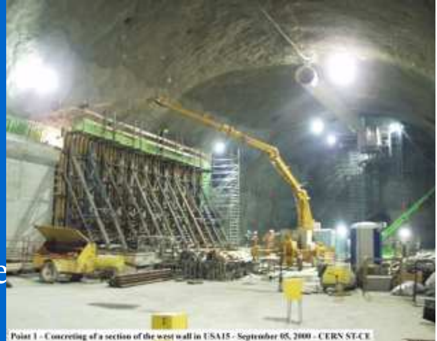
Point 1 - Concreting of a section of the west wall in USA15 - September 05, 2000 - CERN ST-CE
