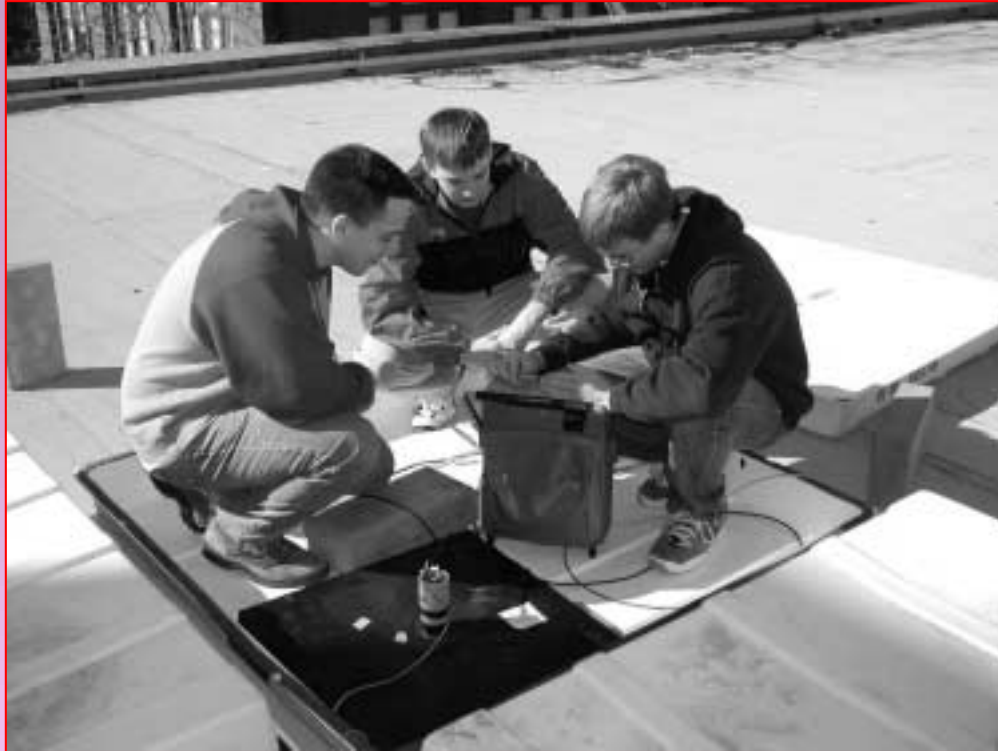
Installation on Physics Department roof, February 2002
